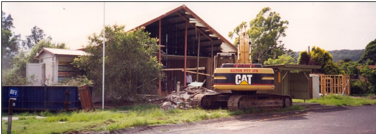
Removal of the projection box which had been pulling at the front wall, was a major achievement.
